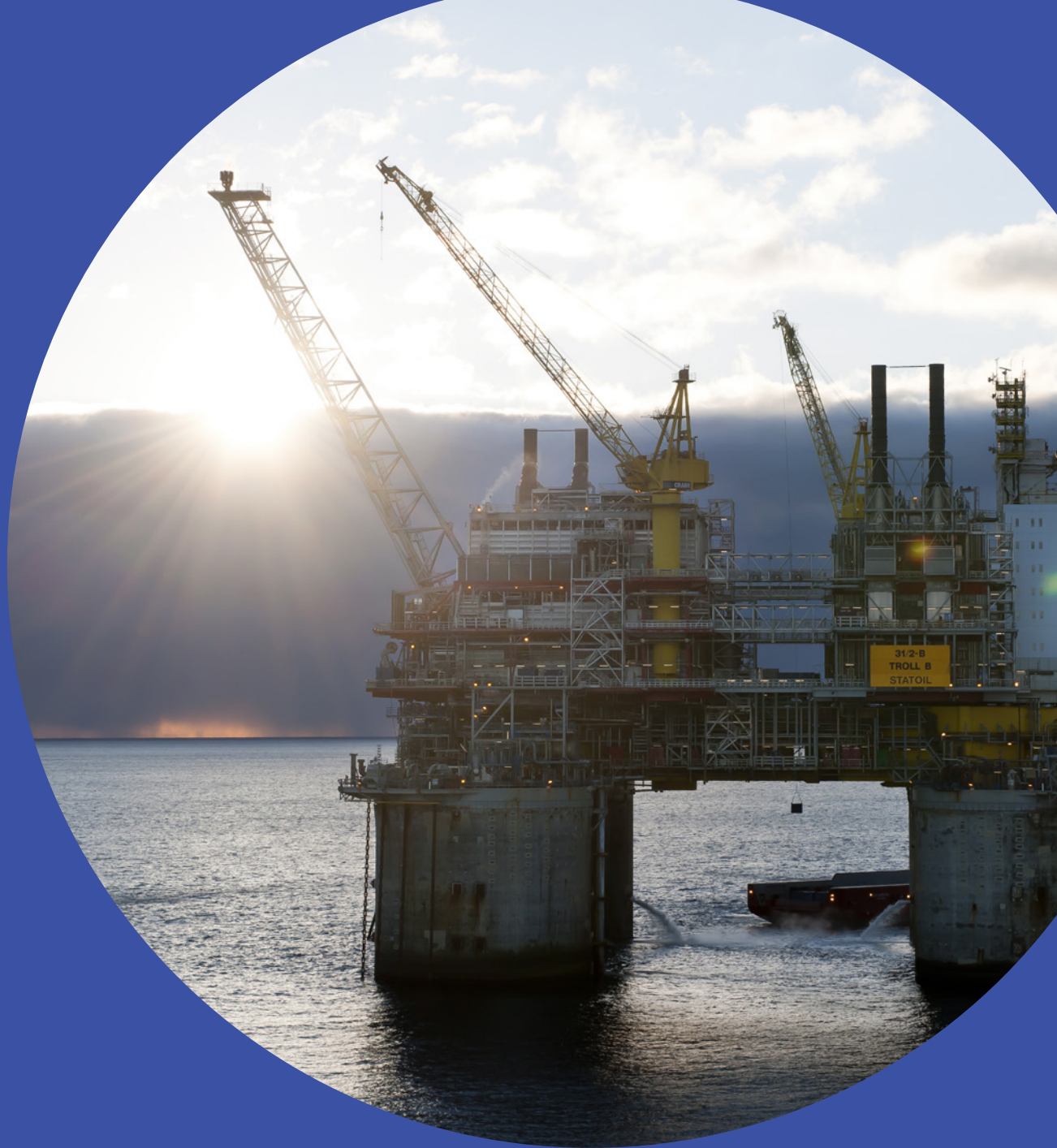
Troll B Photo: Øyvind Hagen, Equinor
